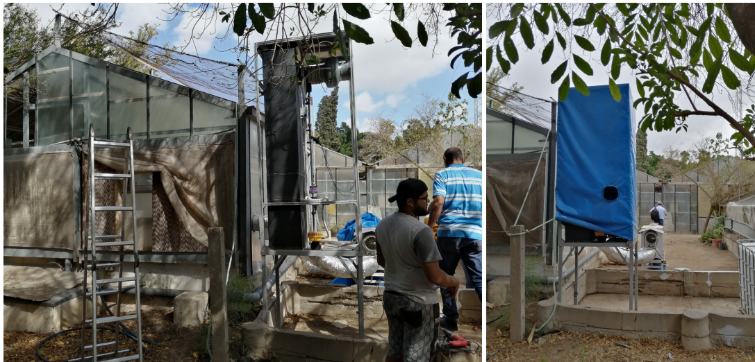
Fig. 15-16 Placement of the absorber on a platform to allow return flow of TCF to the storage (right side of the picture) by gravity
