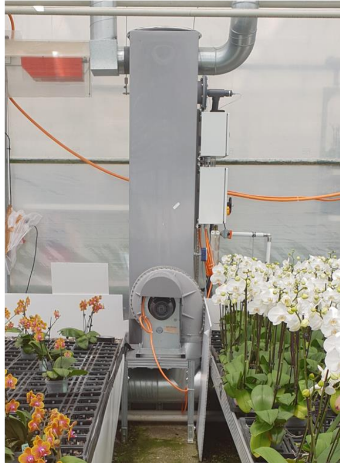
Figure 9. Transparent absorber at ZHAW-lab (left) and the absorber installed in the Swiss demonstrator (right).
