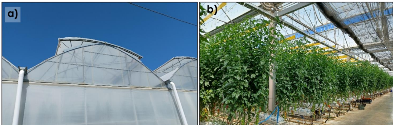
Figure 49. Heated multispan commercial greenhouse (a) and tomato crop in substrate with heating pipes (b) of Sfera Agricola in Italy.
