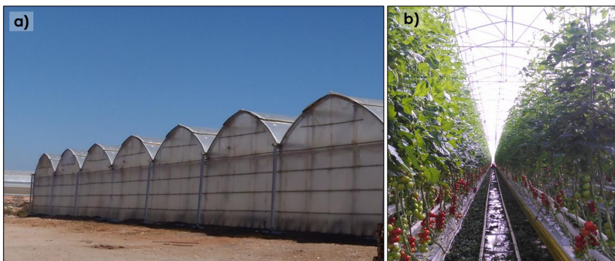
Figure 47. Heated multispan commercial greenhouse with double cover (a) and tomato crop inside (b) of the company Natural Growers in Almería.
