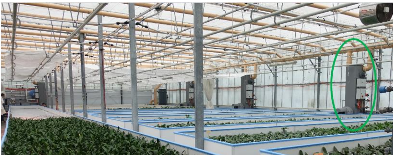
Figure 13. Planting tables in the Swiss demonstrator. In green, the absorber is marked.
