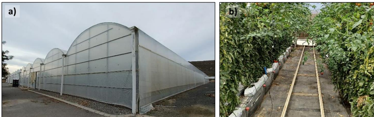
Figure 46. Unheated multispan greenhouse (a) and tomato crop inside (b) in the UAL-ANECOOP Experimental Station in Almería (Spain).
