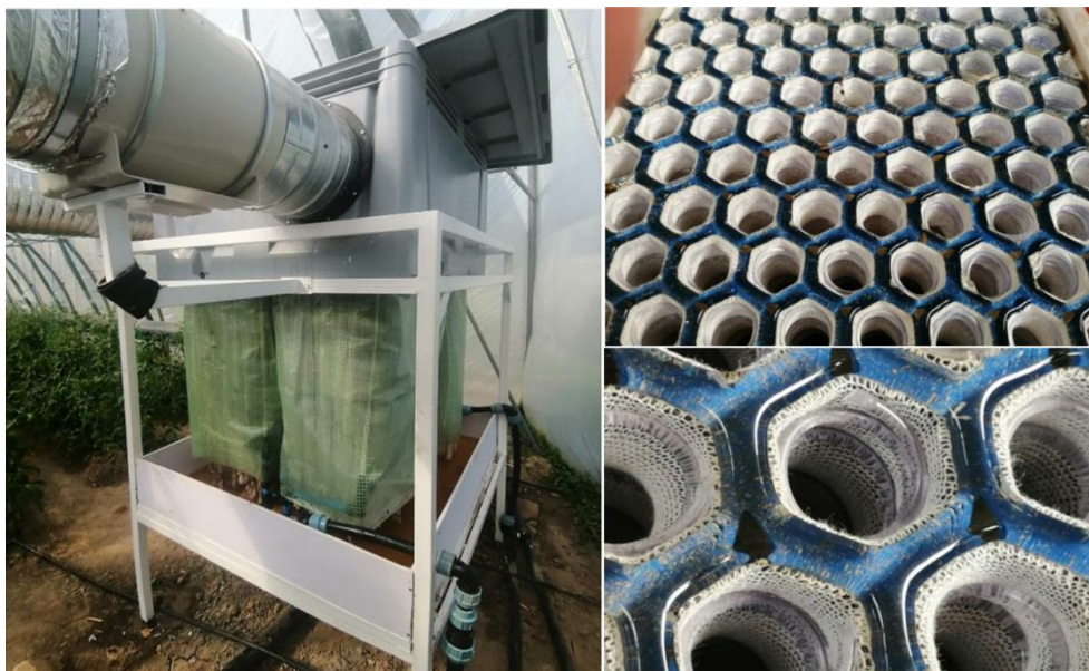
Figure 28. The absorber installed in the Tunisian demonstrator (left) and inside structure of the absorber (right).
