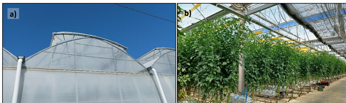
Figure 136. Heated multispan commercial greenhouse of Sfera Società Agricola Srl (a) and tomato crop in substrate on heating pipes (b) in Italy.
