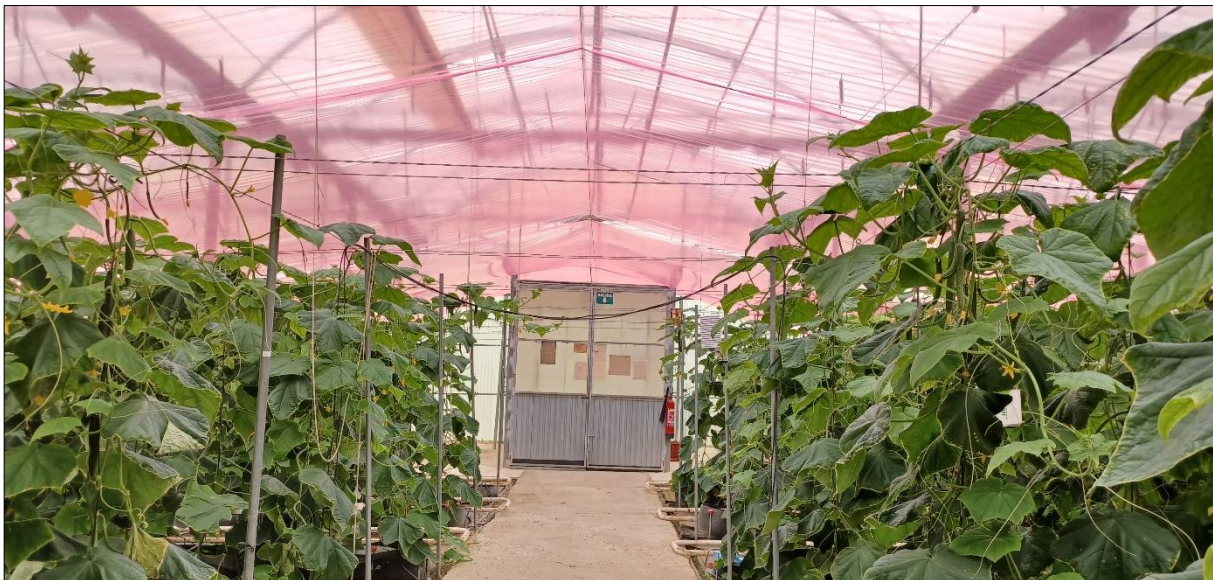
Figure 22. Double roof with a photoconversion of spectrum film inside a multispan greenhouse in Almería (Spain).
