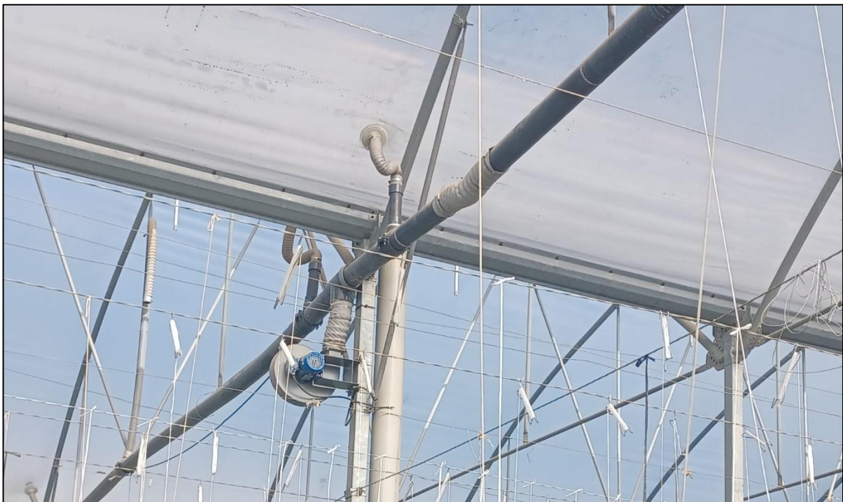
Figure 21. Use of inflated double cover in an unheated multispan greenhouse in Almería (Spain).
