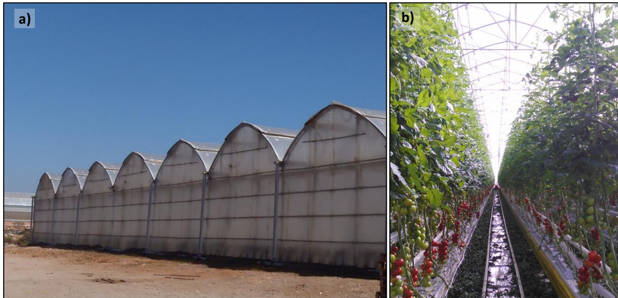
Figure 134. Heated multispan commercial greenhouse with double cover (a) and tomato crop inside (b) of the company Natural Growers in Almería.
