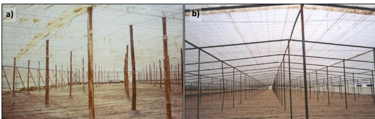
Figure 29. Interior image of elementary greenhouses without roof ventilation, with flat structure and wooden pillars (a) and with gabled structure of metal tubes (b).
