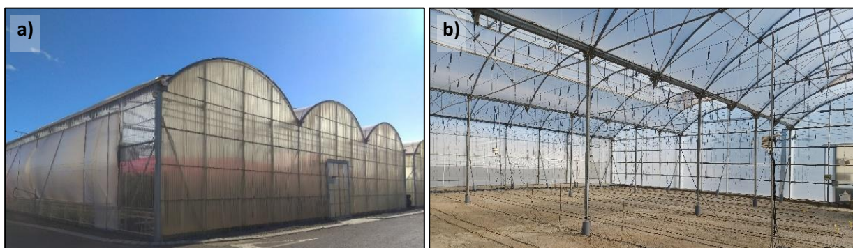
Figure 33. Images of high-tech greenhouses with a multi-tunnel structure of the exterior with rigid polycarbonate front wall (a) and interior with flexible walls (b).
