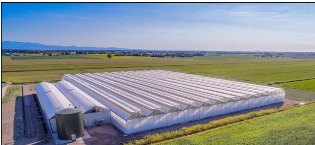
Figure 122. Multispan greenhouses in Italy (ILS, 2023).
