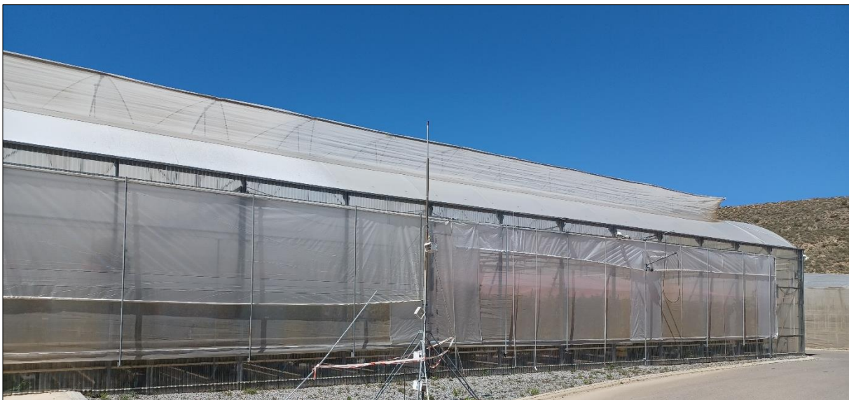
Figure 15. Multispan greenhouse in Almería with increased side openings.
