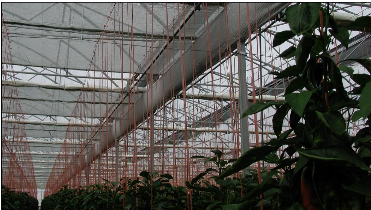
Figure 23. Thermal screen inside a Venlo glasshouse with a pepper crop in Almería (Spain).
